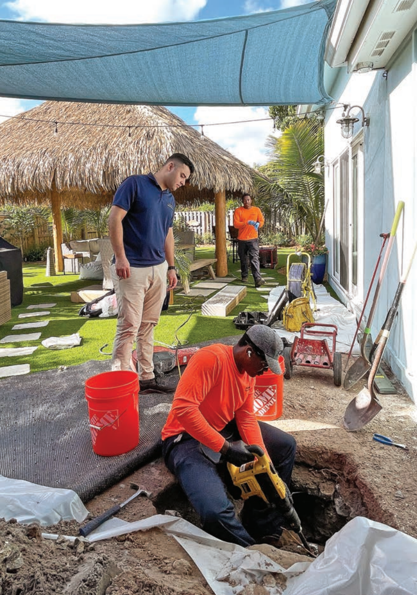
▲ Jones breaks up rock to expose a pipeline in the access pit.
